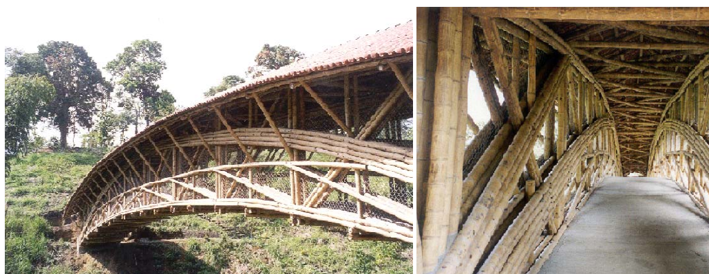
Figure 4- 32 Bamboo bridge in Pereira with 52 meters span designed by Jörg Stamm, 2001 (ref. Jörg Stamm)
