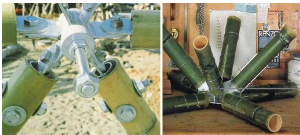
Figure 4- 36 Bamboo connections by Shoji Yoh (left) and Renzo Piano (right) (ref. Shoji Yoh + Architects; Renzo Piano Building Workshop)
