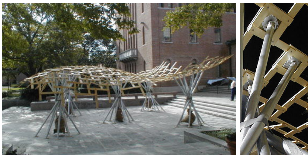
Figure 4- 22 Bamboo Roof at Rice University in Houston, USA, 2002/03, Shigeru Ban Architects (ref. Shigeru Ban Architects)
