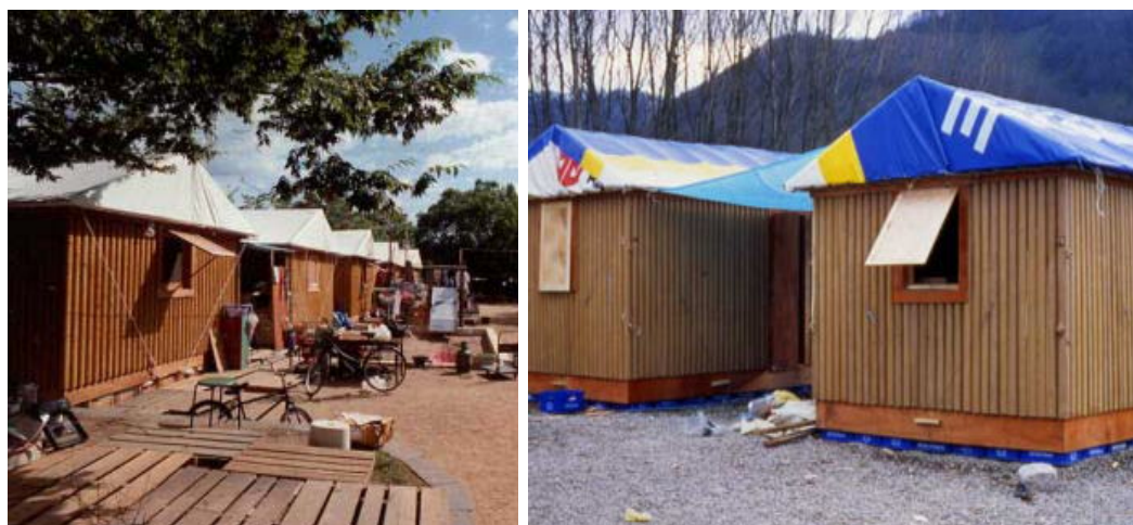
Figure 4- 58 Paper log house for refugee in Kobe, Japan 1994 (left) and in Kaynasli, Turkey 2000 (right) by Shigeru Ban (ref. Shigeru Ban Architects)
