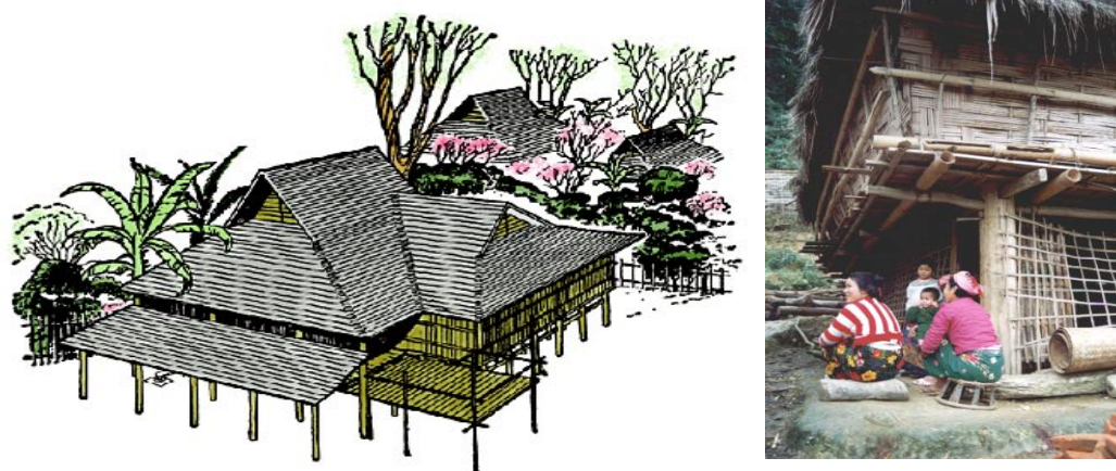
Figure 2- 17 Bamboo Architecture "GanLan" style in South China
