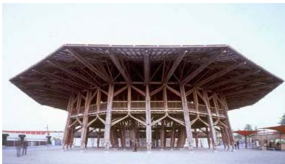
Figure 4- 31 Zeri Bamboo Pavilion in Expo2000 Hanover designed by Simón Vélez
