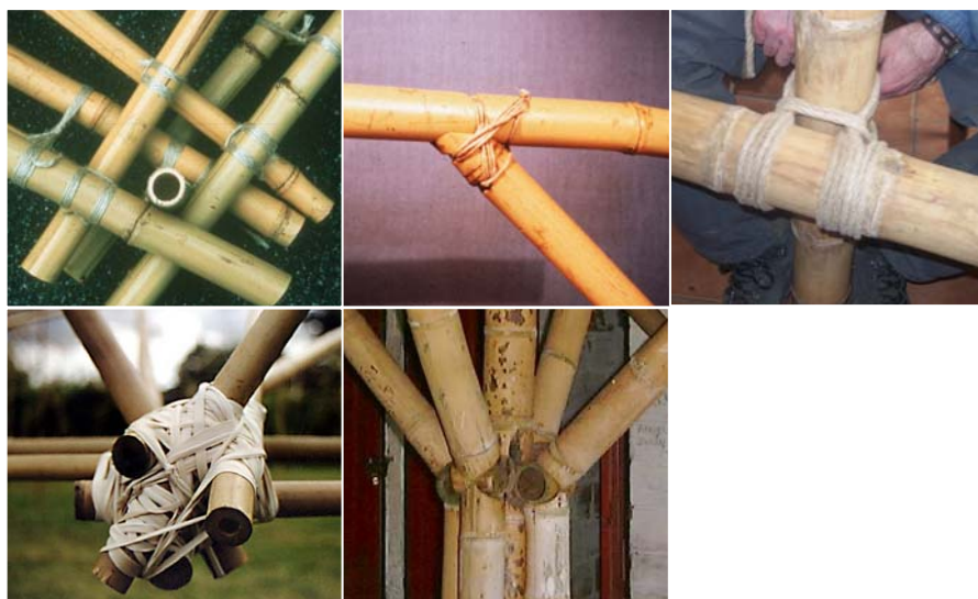
Figure 4- 26 Some bamboo connections
