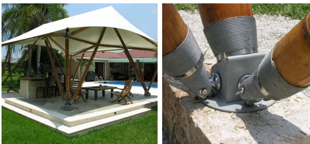
Figure 4- 34 Bamboo pavilion and its connection by Koolbamboo
