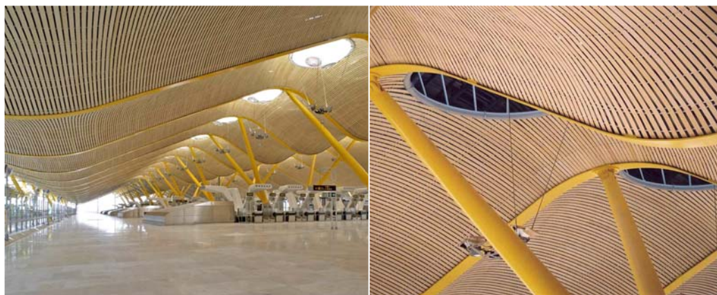
Figure 4- 23 Bamboo Roofs in the Madrid Barajas Airport by Richard Rogers Partnership and Estudio Lamela, 2006 (ref. Amparo Garrido and Richard Bryant/arcaid.co.uk)
