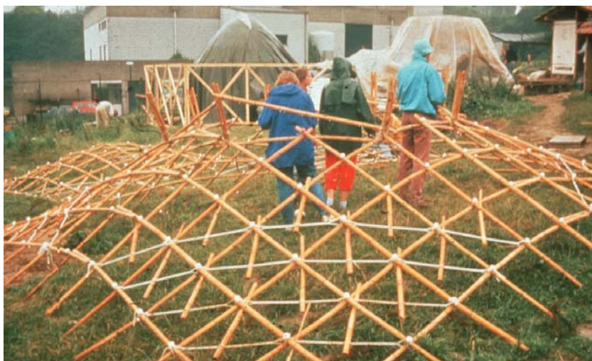
Figure 4- 29 Bamboo grid shell structure by Baier in Aachen
