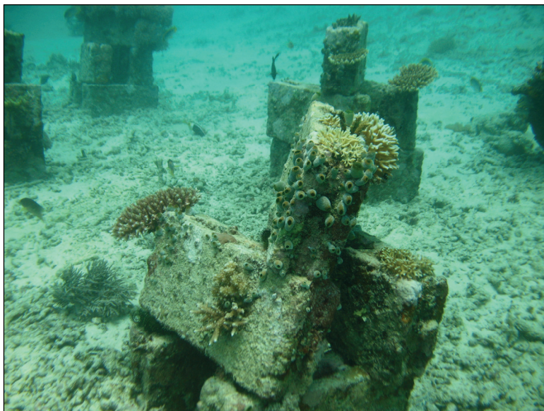
Figure 4.18: 30 months after construction, a diverse epibenthic community consisting of soft and hard corals, sponges, tunicates and other organisms had developed on the concrete structures, as shown here on Gangga.
